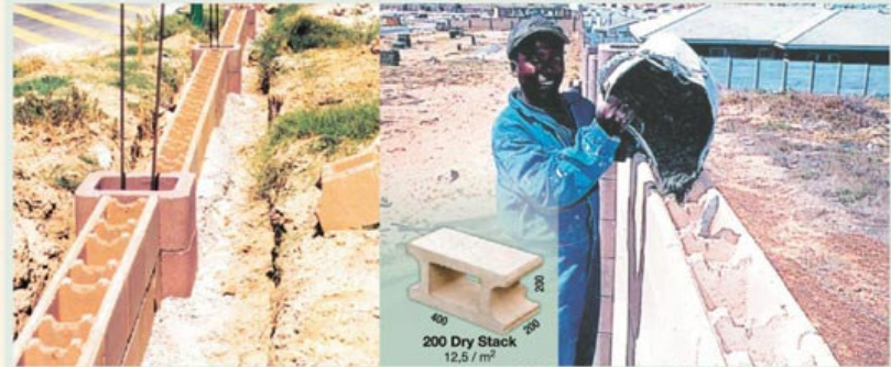
First row to be levelled in mortar on the concrete slab to ensure 100% level.
